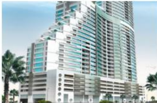
Al Jaber Tower
