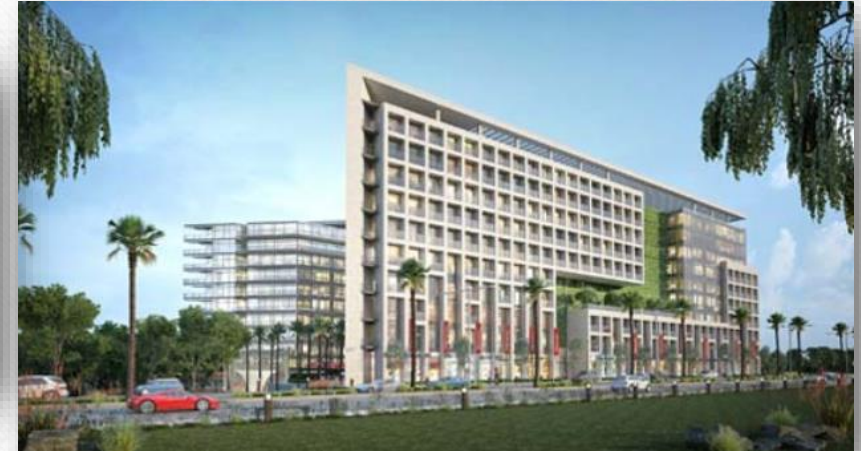
SDW4-C1 Park View Bldg.
